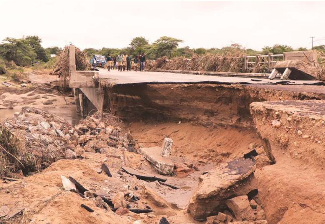
Nkankezi Bridge (connecting Zvishavane and Mbalabala) washaway due to Cyclone Dineo induced floods
